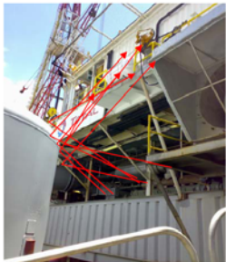
Diagram 8: Noise path from EMDs.
